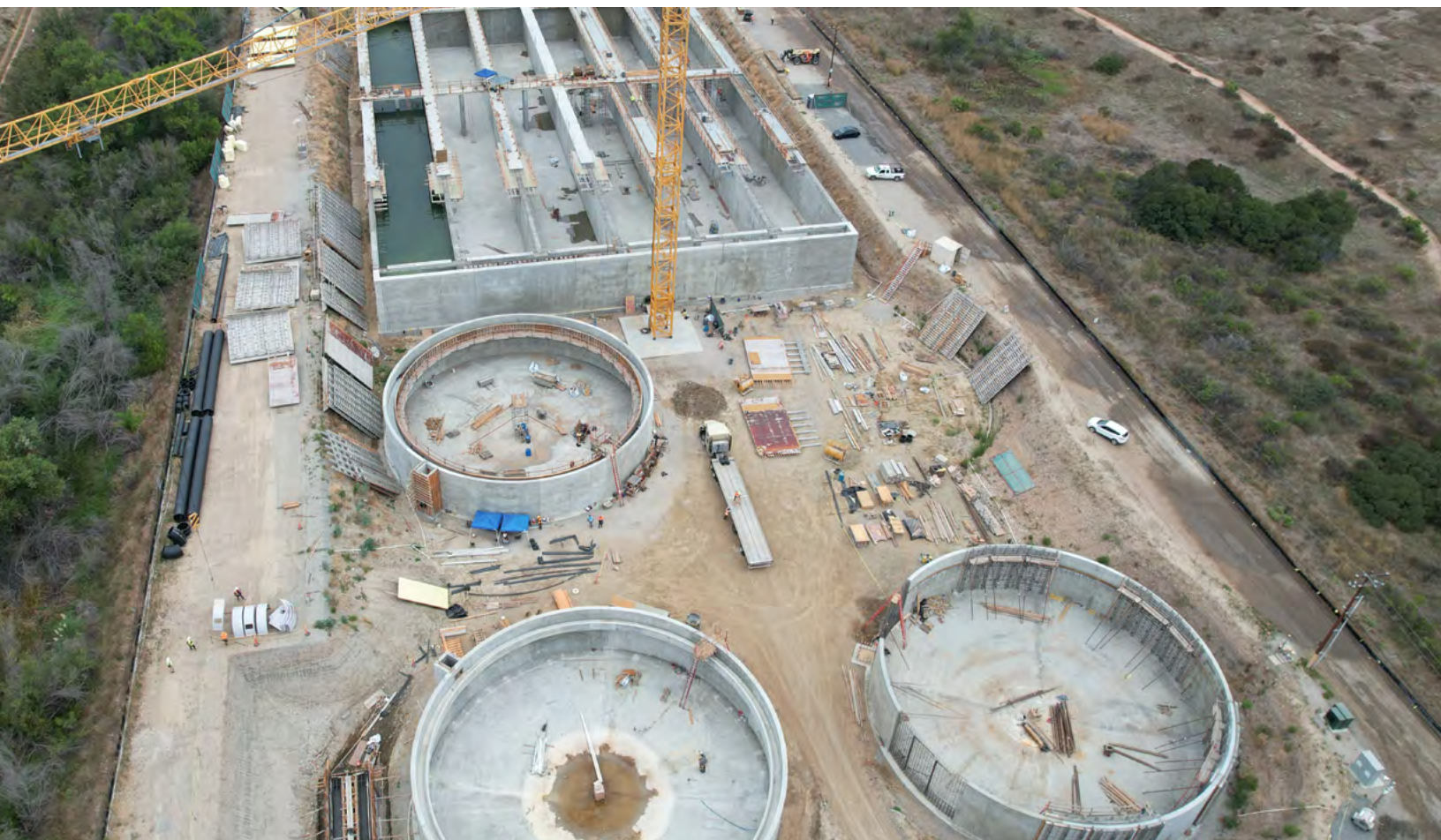
Construction of the East County Advanced Water Purification Project, a Local Resources Program project in the service area of the San Diego County Water Authority.
