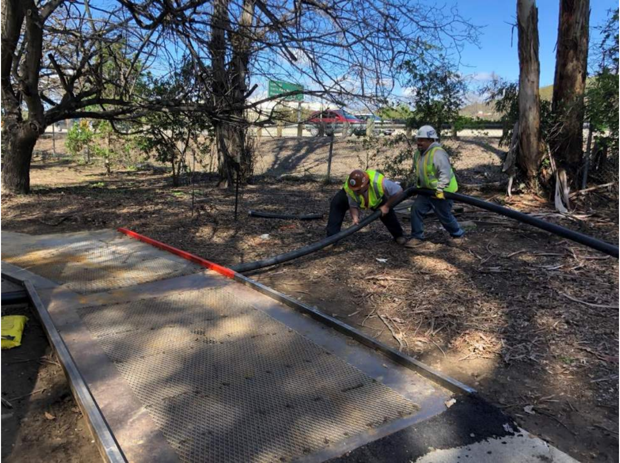
Site Photo 13 Feed Piping Installation
