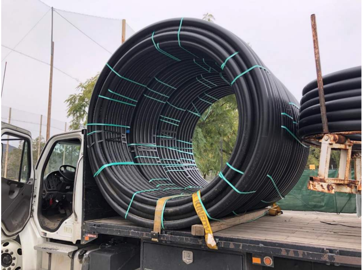
Site Photo 4 Flexible Tubing for Feed Water
