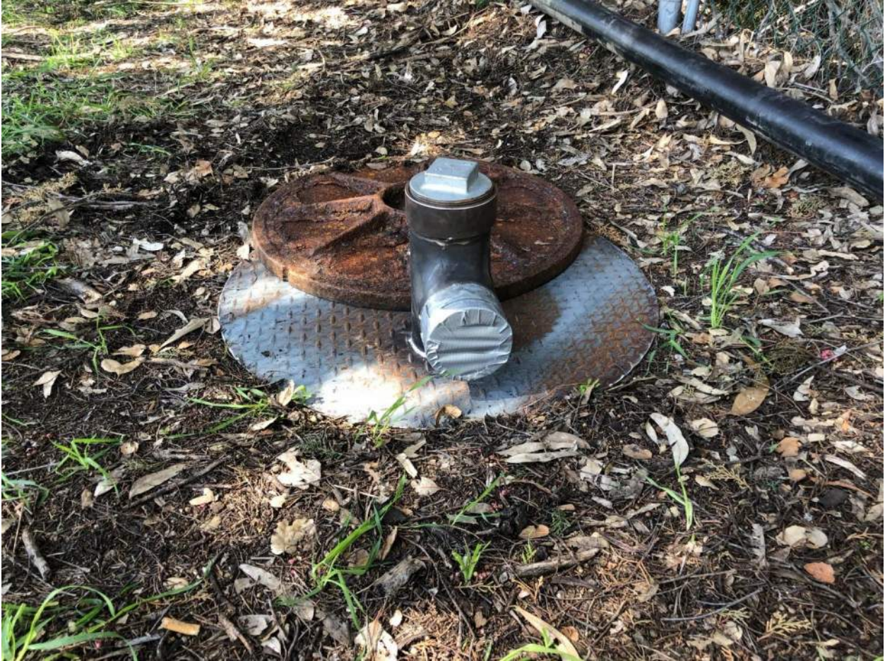
Site Photo 11 Sewer Connection
