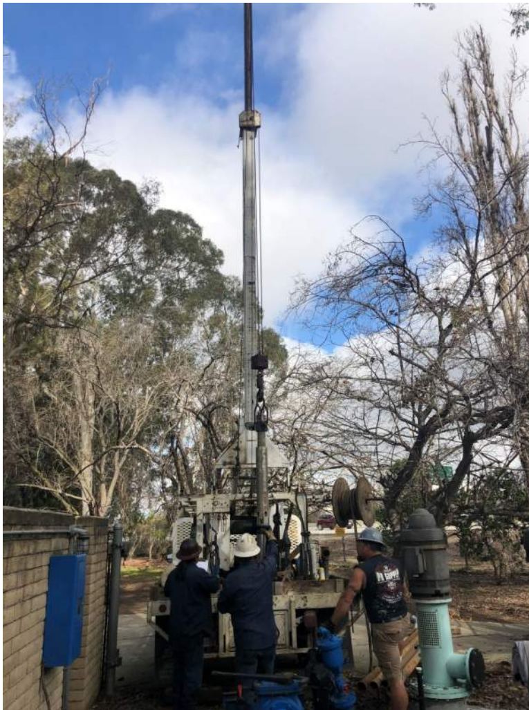
Figure 19: Well Pump Installation
