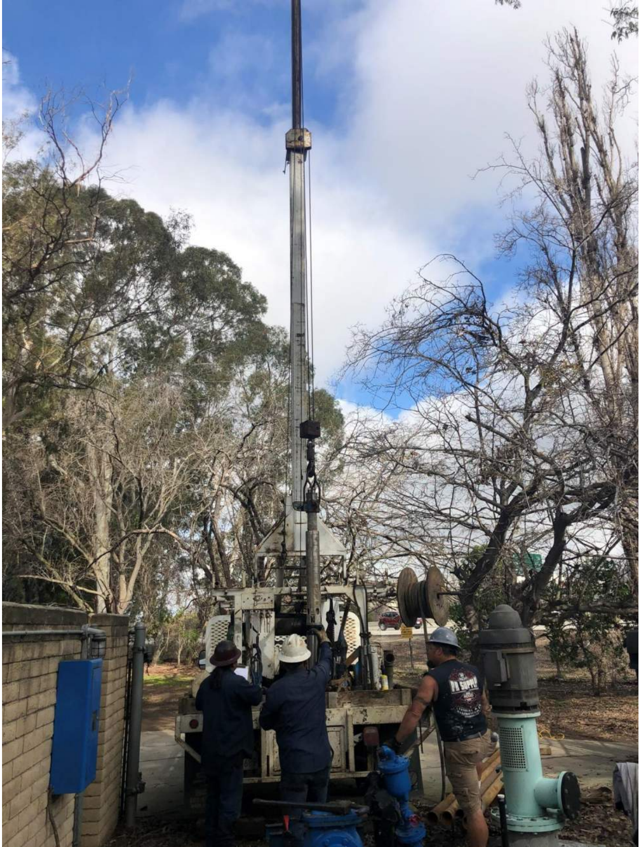
Site Photo 6 Well Pump Installation
