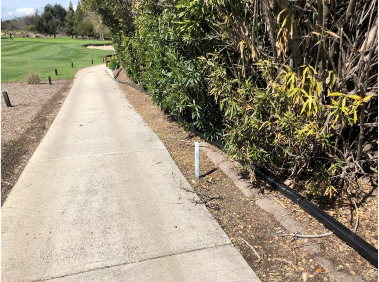
Site Photo 8 Feed Tubing
