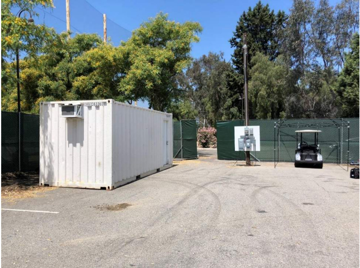
CCRO System Photo 2 Container
