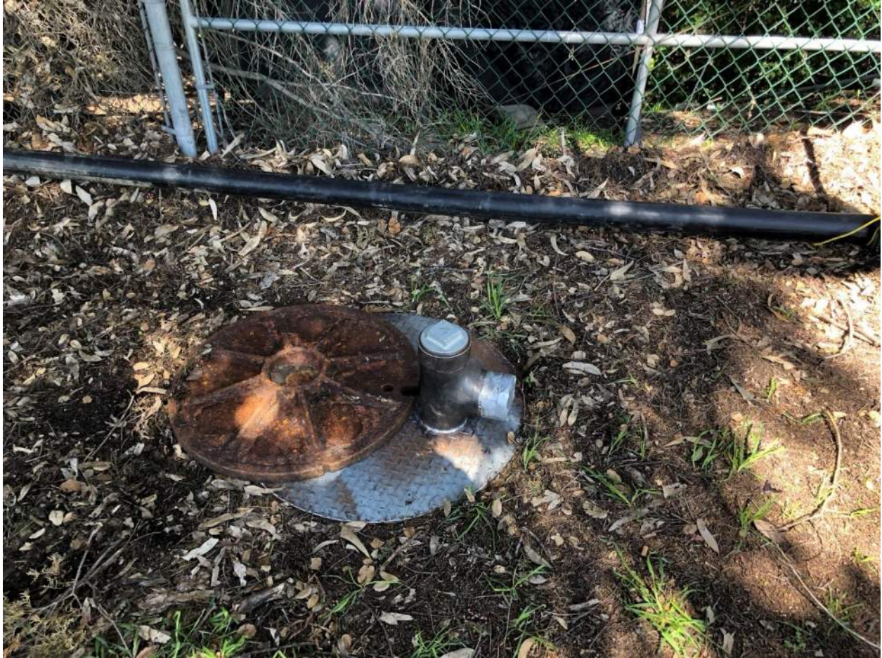
Site Photo 12 Sewer Connection
