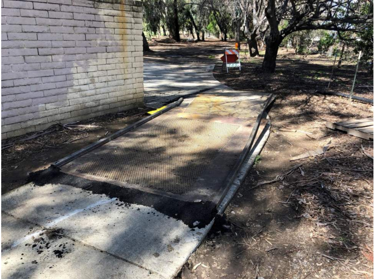
Site Photo 10 Temporary Golf Cart Ramp
