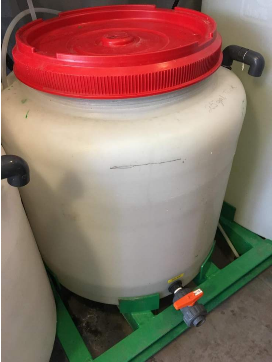
CCRO System Photo 5 Chemical Drums
