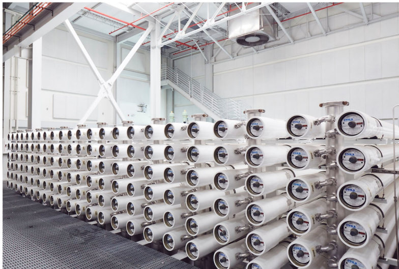
Figure 8-3. A 5-MGD RO Unit at OCWD AWPf Equipped with Hydranautics ESPA2-LD Membranes.
