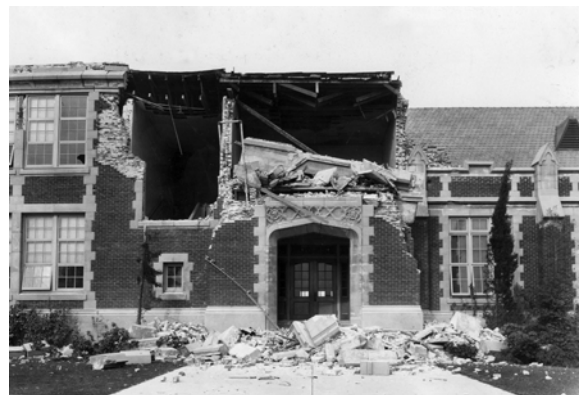
The 1933 M6.7 Long Beach earthquake took place on March 10 at 5:54 P.M. Damage to buildings was widespread and between 115 and 120 people died. The earthquake highlighted the need for earthquake-resistant design for structures in California.
