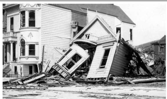
The 1906 M7.8 San Francisco earthquake struck the coast of Northern California at 5:12 a.m. on April 18. Severe shaking was felt from Eureka on the North Coast to the Salinas Valley. Broken gas lines resulted in fires that lasted for several days due to a lack of fire supply. As a result, about 3,000 people died and over 80% of the city of San Francisco was destroyed.
