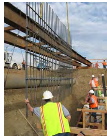
Metropolitan construction crews
