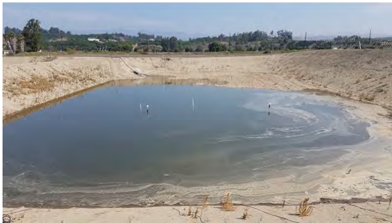
Figure 21. The filling of Pond 10 with 407k gallons (1.5 AF). The pond was never filled due to the high infiltration rates that were similar to the pump outflow rates.
