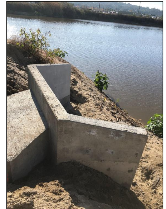
La Palma/Richfield Diversion and Infiltration Project
